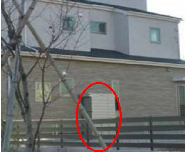
A. Installation at house
